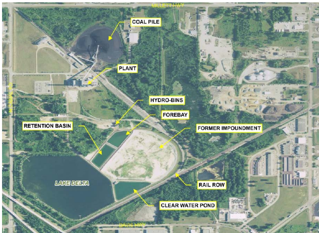
Figure 2. Erickson Power Station Site Configuration
